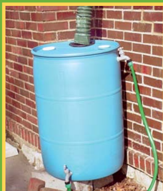
Finished rain barrel at work
